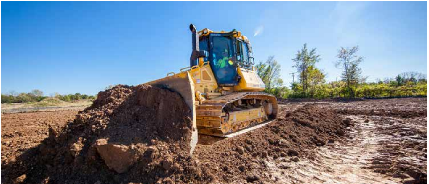
A Komatsu D51PXi hogging on the Old Morrison jobsite. “We see tremendous value in utilizing an i-machine for installation of the laydown yard,” commented Sykes. The site consists of a 60,000 sq. ft. service center and a 170,000 sq. ft., stone laydown yard for AEP crews. The project also entails 5,000 lf. of waterline, 3,700 lf. of storm and 1,200 lf. of sanitary work.
